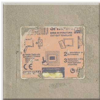
2 Nanesite malter Apply the mortar
